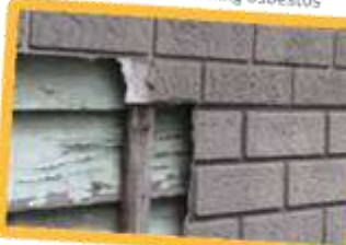
External cladding containing asbestos
