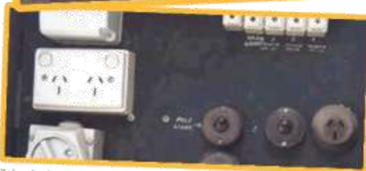
Zelemite backing board to an external switchboard
