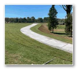
Old College Road, Gatton - Upgrade Existing Concrete Footpath (Gaul Street to Park Lane) This project involved the construction of 65 metres of new concreted footpath to the south side of Old College Road. Works were completed on 8 January 2021.
