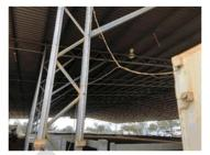
Figure 14 and 15: Existing cables strung without adequate support.
