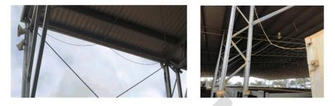
Figure 14 and 15: Existing cables strung without adequate support.
