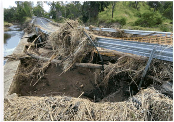
147 locations that require rock fill to protect remaining structures, this is primarily around concrete flood way structures that have been damaged due to fast flowing, high water.
