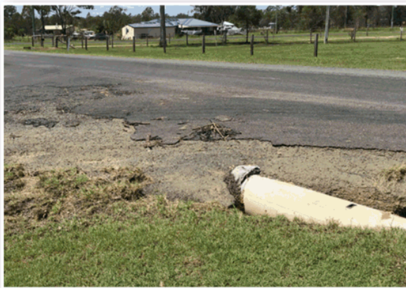
20 pipes that have been identified with separation between the pipe units
