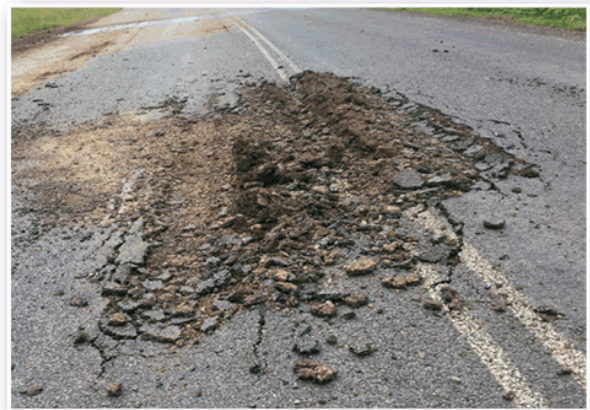
103 locations where the pavement has been damaged from the flood event, this can be caused due to water washing over the road and damaging the surface, in other incidents it will be damage from the pavement being saturated and vehicular movement on the roads causing pavement failures
