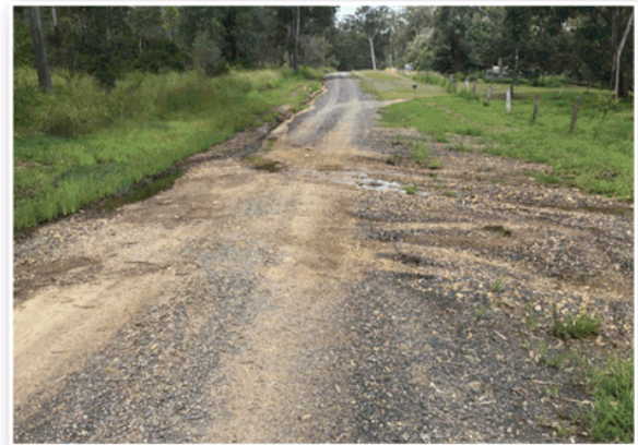
145 roads that requires grading due to damage caused by the February rain event.
