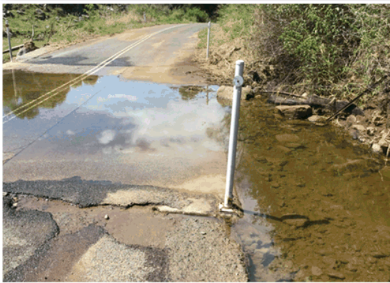
120 drainage structures that require the removal of silt and rubble to re-establish a functioning culvert/pipe.
