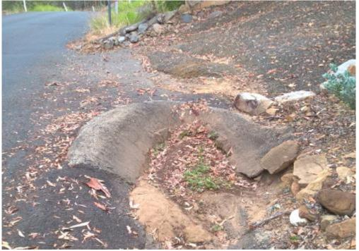
Figure 3: Blocked upstream driveway pipe
