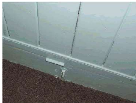
Ventilation flaps at skirting level
