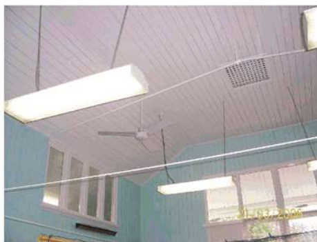
Ceiling vents and tie rods
