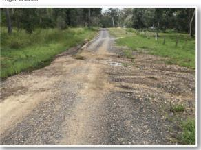
145 roads that requires grading due to damage caused by the February rain event.
