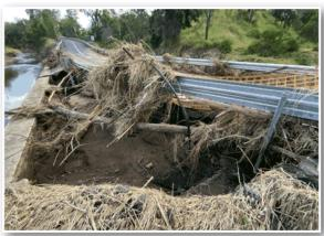
147 locations that require rock fill to protect remaining structures, this is primarily around concrete flood way structures that have been damaged due to fast flowing, high water.
