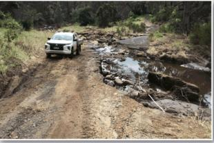
251 locations that requires fill to be placed around structures and road formation to protect existing assets and to provide a safe path of travel.
