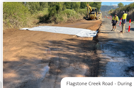
Flagstone Creek Road - During
